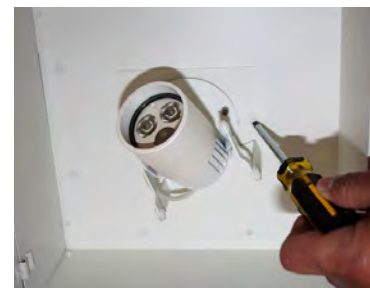
9. If applicable Push up Light Fixture through top housing access and screw Fixture onto top housing access.
