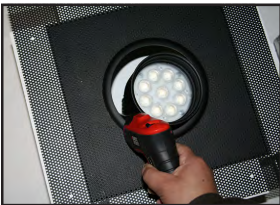
12. Screw Fixture onto top housing access.
