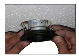
**9**. Push Fixture into opening. There will feel spring resistance and fixture will snap in place.
