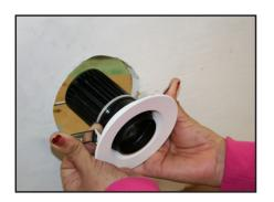
8. Push springs back and Insert fixture and springs into opening.
