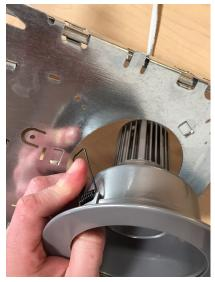
2. Fold up spring clips and push fixture opening. Then release clips.
