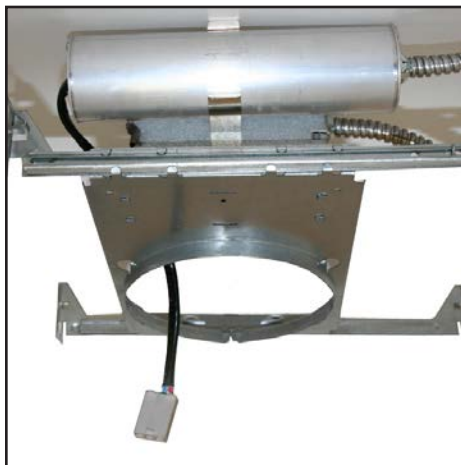
5. Pull Transformer Pig Tail through opening
