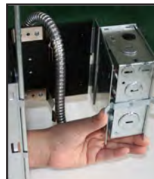
C. Snap Close the J-Box and secure Ballast inside holding clips and replace side panel access cover.
