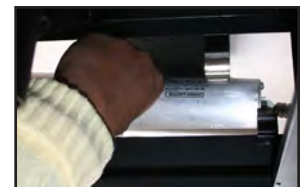
C. Snap Close the J-Box and secure Ballast inside holding clips and replace side panel access cover.
