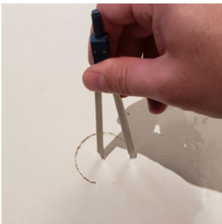
1. Score a 1 \frac{7}{8} " (1.875") hole in the drywall.
