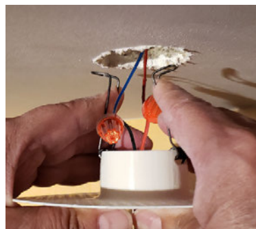
5. Fold back spring clips and push into the hole.
