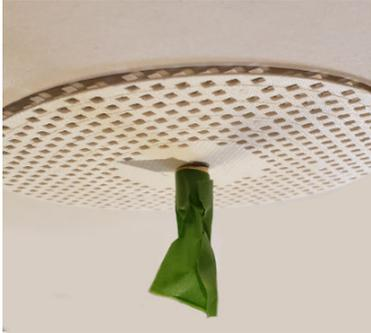
6. (Optional) Wrap coupling and female end of wire with tape to protect from spackle.
