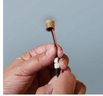
10. Connect male end of wire from the back of the fixture to the female end sticking out of the coupler.
