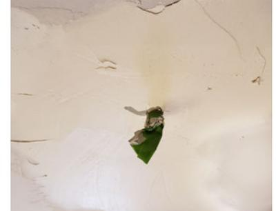
7. Apply a layer of spackle and allow to dry completely. Reapply layers as necessary.
