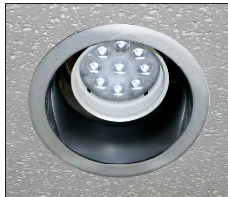
10. Restore electrical Power and check the operation of your new CLARTÉ light fixture.
