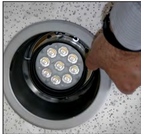
8. Insert LED fixture into opening and press firmly into the clips until securely in place.
