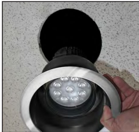
8. Insert LED fixture into opening and press firmly into the clips until securely in place.
