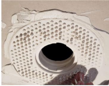
6. Align the screen hole with the hole in the ceiling and firmly press the screen into the wet joint compound. Make sure the joint compound comes out through the mesh holes and that the mesh is sitting flush against the ceiling.
