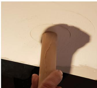
10. Wrap the fixture to protect the finish then install fixture by turning COUNTER-clockwise and it will click when in place.
