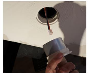
9. Connect wire from inside ceiling to back of the fixture.
