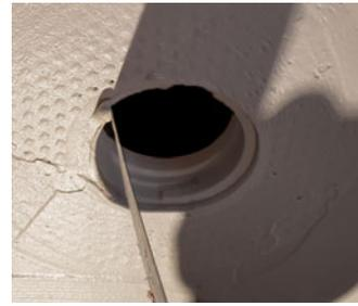
8. Remove excess joint compound from the opening to ensure the fixture will install and fit properly. Allow spackle to dry.
