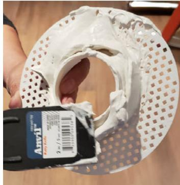
4. Generously apply joint compound to the back of the screen along the outside collar of screen opening. This will ensure any gap around the hole cutout will be filled. There should be enough applied to fill in any gaps around the hole and will push through inside the ceiling (see picture 2).
