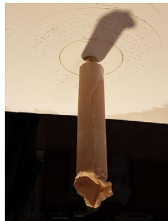
11. Slightly unscrew fixture so there is a gap between the ceiling and back of the fixture.
