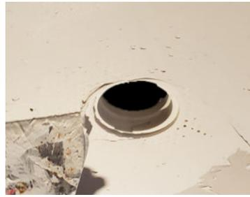
7. Apply as much joint compound as needed and begin to smooth out the surface.
