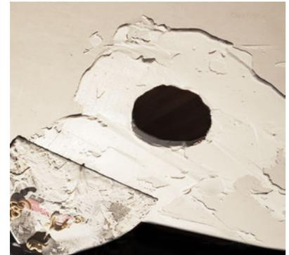
5. Apply joint compound around the hole in the ceiling.
