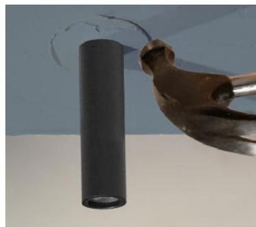
15. To remove fixture for servicing use a hammer to tap around the perimeter of where the hole is until the trim is free.
