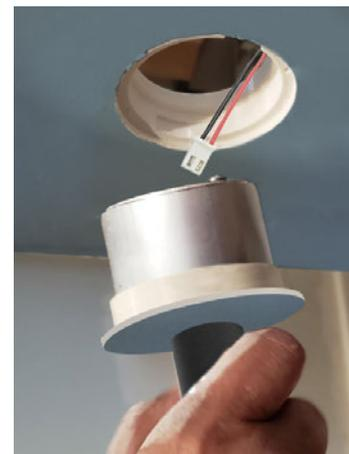
16. Firmly turn the fixture CLOCKWISE to remove. Minimal damage to the painted plate makes re-installation a breeze.
