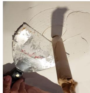
12. Reapply layers of joint compound as necessary.
