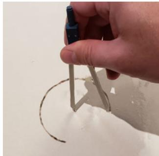
2. (If you don't have a 3" hole cutter bit) Score a 3" hole in the ceiling and use a hand saw to cut out the hole.
