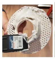
4. Generously apply joint compound to the back of the screen along the outside collar of screen opening. This will ensure any gap around the hole cutout will be filled. There should be enough applied to fill in any gaps around the hole and will push through inside the ceiling (see picture 2). Plug style may differ.
