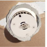
5. Apply joint compound around the hole in the ceiling.
