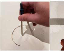
2. (If you don't have a 3" hole cutter bit) Score a 3" hole in the ceiling and use a hand saw to cut out the hole.
