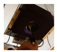
4. Push up light fixture into top housing to access screws and screw fixture into top housing (2 screws, use magnetic tip screwdriver).
