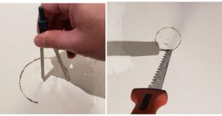
2. (If you don't have a 4" hole cutter bit) Score a 4" hole in the ceiling and use a hand saw to cut out the hole.
