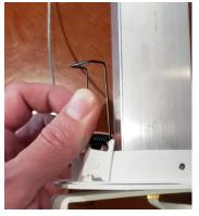
4. Fold up springs clips and push fixture through hole then release clips.
