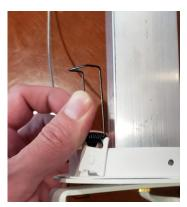
5. Fold up springs clips and push fixture through hole then release clips.
