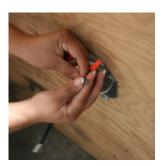
1.Install standard j-box. Make wire connections. Black with black, white with white and ground with ground.
